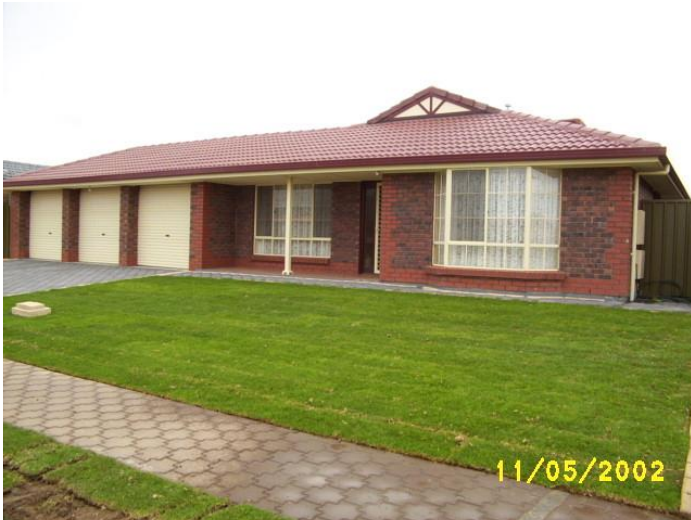
Built this Luxury House in Adelaide 2002 did all the Improvements myself
